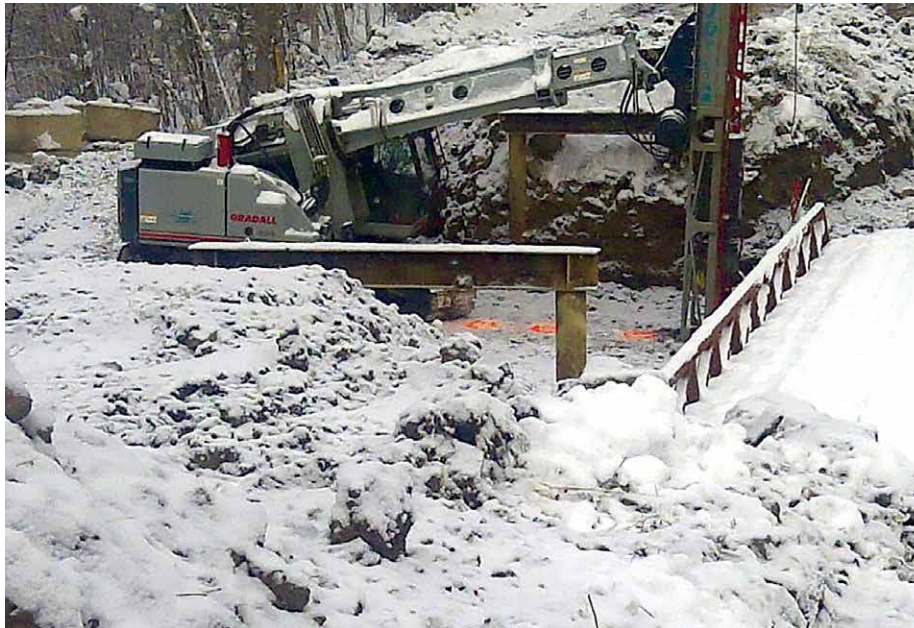
Drilling through permafrost in Canada’s Northwest Territories.
