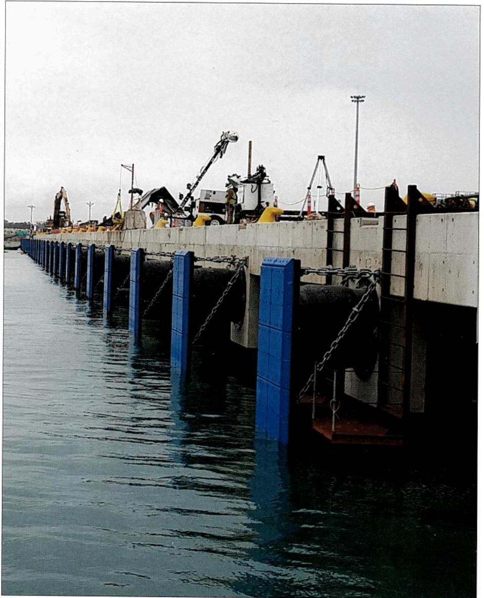
Last year, the U.S. office of SFT delivered 55 CSS 1450 Cell Fender Systems (G2.0), 8 nos. CSS 630 Cell Fender Systems and several Bollards to the new APM container terminal in the Caribbean port of Moin, Cost Rica
