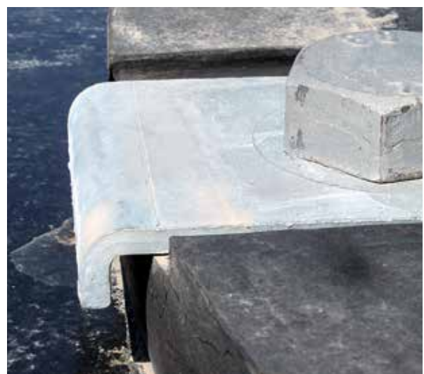
Maasvlakte II | Rotterdam | The Netherlands
