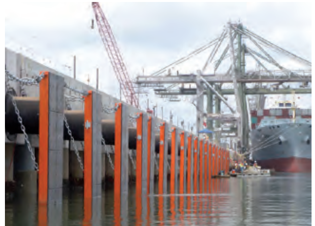
Barbour's Cut Container Terminal | Houston, TX | USA
