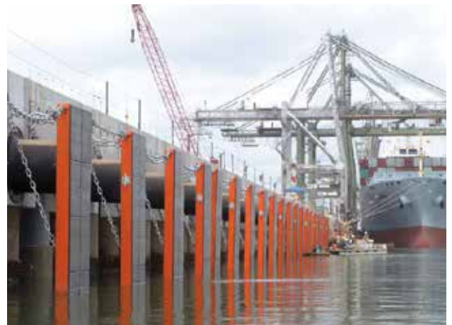
Barbours Cut Container Terminal | Houston, TX | USA
