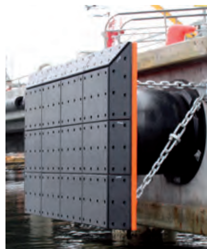
Chemical Product Jetty | Stenungsund | Sweden
