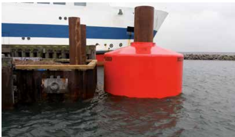
Ferry Terminal | Sejerø | Denmark
