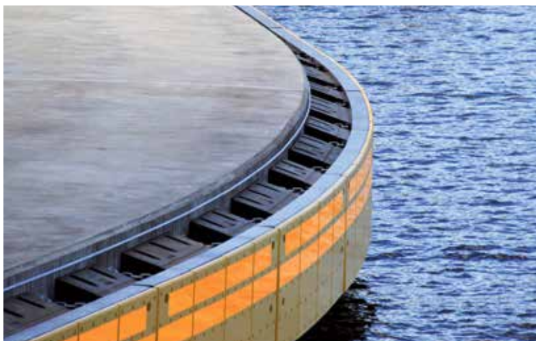
Bridge Protection Guidewall | Stockholm | Sweden
