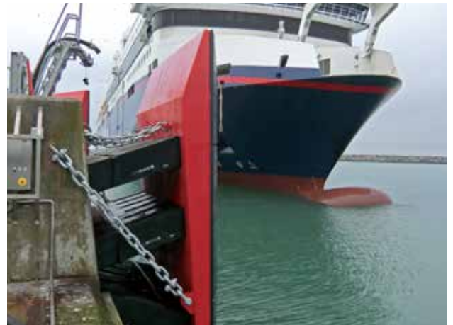
Ferry Terminal | Hirtshals | Denmark
