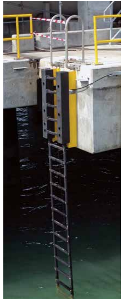
IDPT Jetty 1 | Johor | Malaysia
