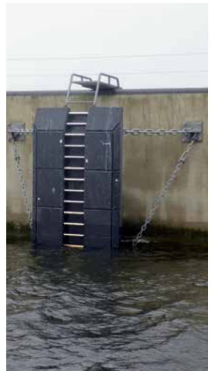
Maasvlakte II | Rotterdam | The Netherlands
