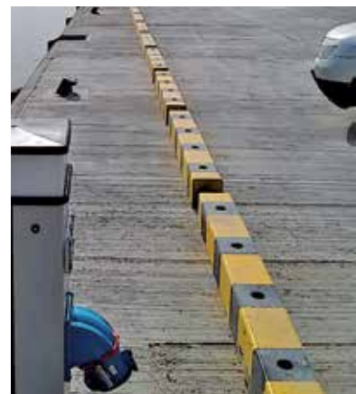
Southern Quay Wall | Simaisma | Qatar
