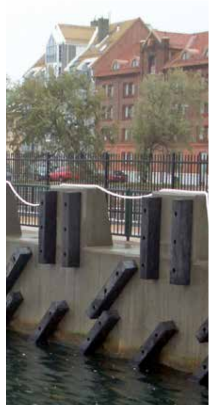
Ferry Terminal | Landskrona | Sweden
